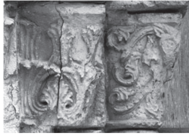
Catenoy west portal
