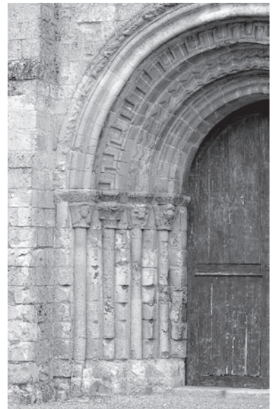
Lavilletterte west portal
