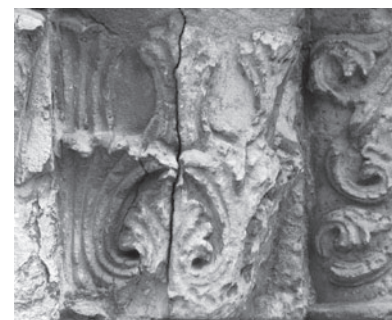
Catenoy west portal
